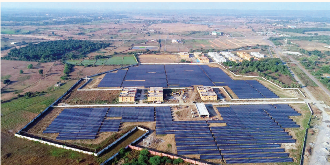
10 MW Solar Power Plant in premises of STPP
